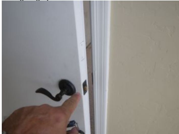
Strike plate needs adjustment to properly secure the door. @ single car garage
