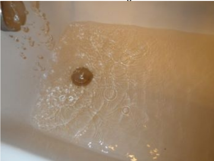
When running cold side water at all water using devices there is heavy rusty water, since it's only the cold side it's possible this can be a water softener issue, Recommend a Licensed plumber evaluate and repair. It's also possible the water softener will need flushing and sanitized.
