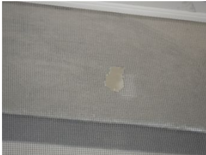
Torn screen at single car garage window, this will need to be re screened.
