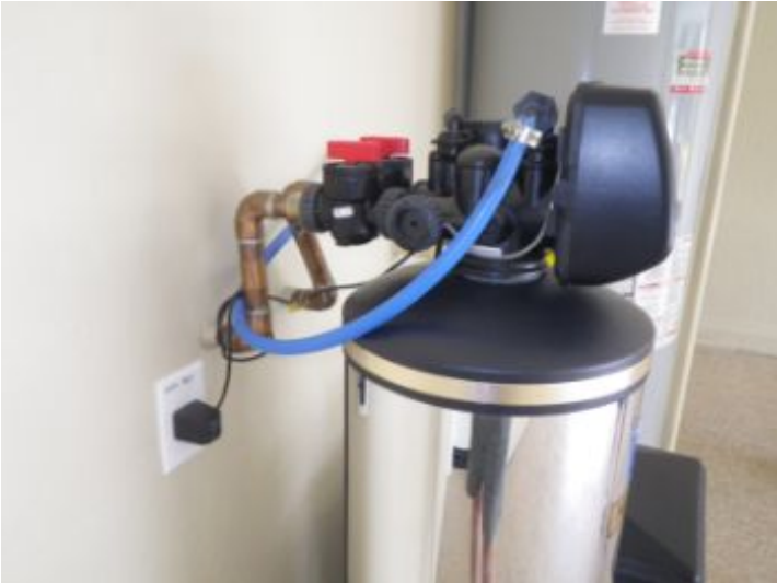
When running cold side water at all water using devices there is heavy rusty water, since it's only the cold side it's possible this can be a water softener issue, Recommend a Licensed plumber evaluate and repair. It's also possible the water softener will need flushing and sanitized.
