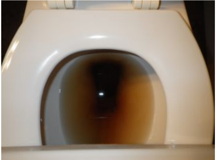
When running cold side water at all water using devices there is heavy rusty water, since it's only the cold side it's possible this can be a water softener issue, Recommend a Licensed plumber evaluate and repair. It's also possible the water softener will need flushing and sanitized.
